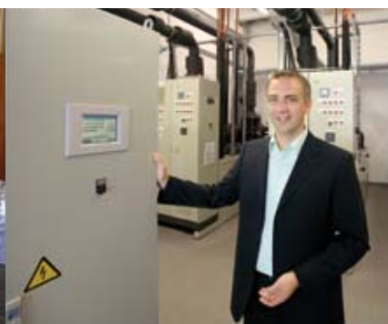
Jörg Missling, head of facility management at arvato systems, ensures optimal energy supplies.
